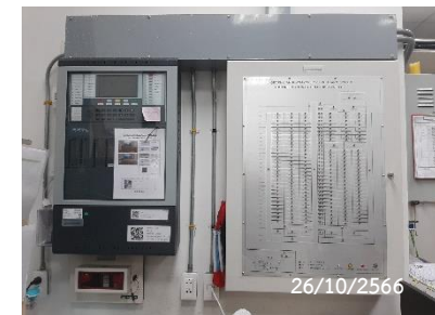
Graphic Annunciator Fire Alarm System
