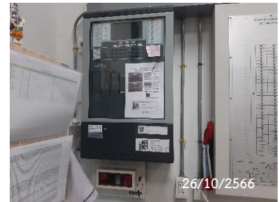
Fire Alarm Control Panel
